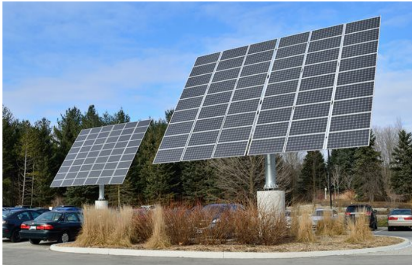
Figure 2. Solar panels mounted on poles with trackers. (image credit Wikimedia Commons user Raysonho)
