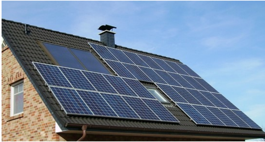
Figure 1. Fixed solar panels on the roof of a house.
