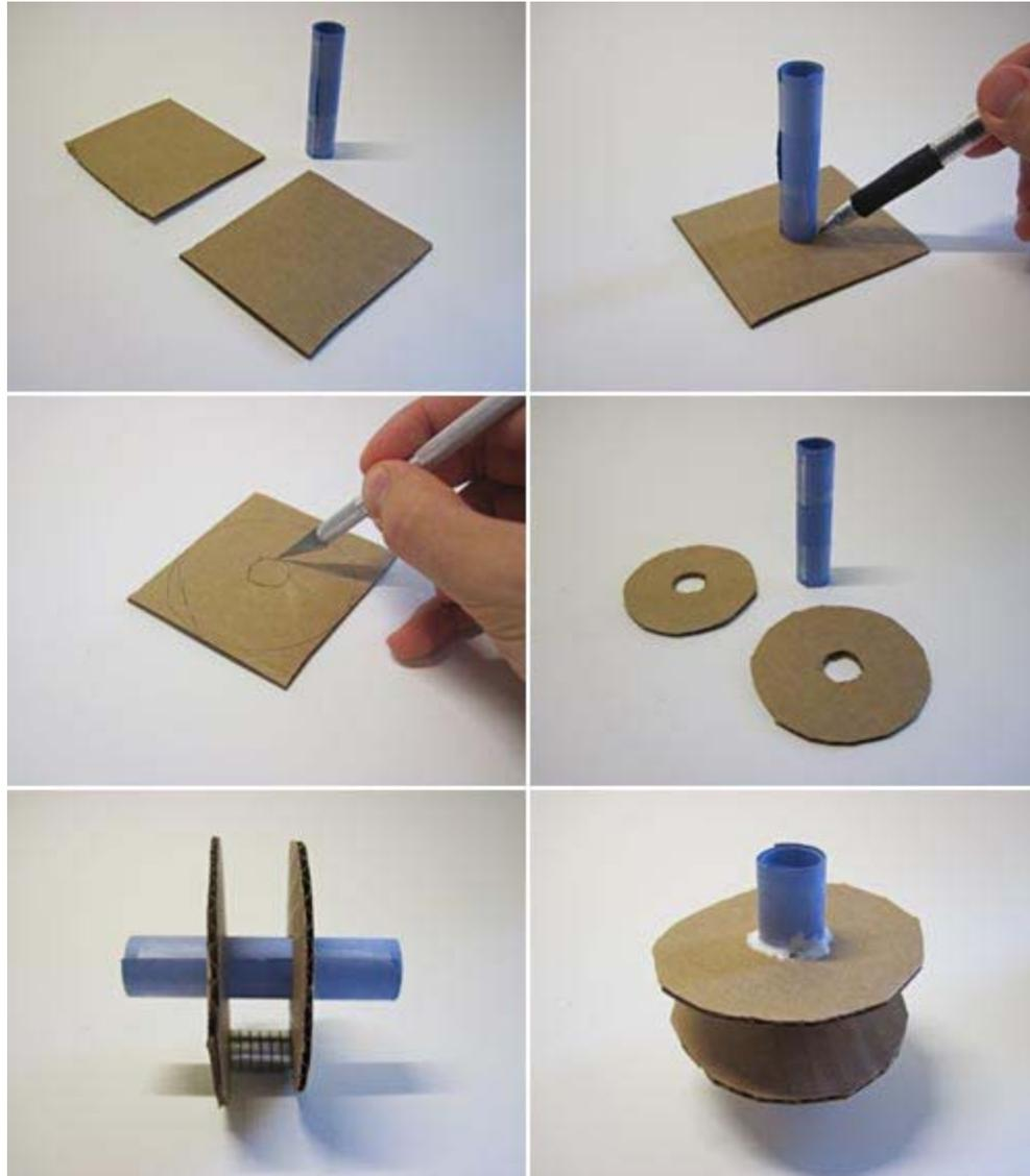
**Figure 5.** Cut out cardboard circles and glue them onto your coil form (the larger card stock tube), as shown here. *Note:* The bottom left image shows the stack of magnets so you know how far apart to space the cardboard pieces — the magnets will not actually stay in this position.
